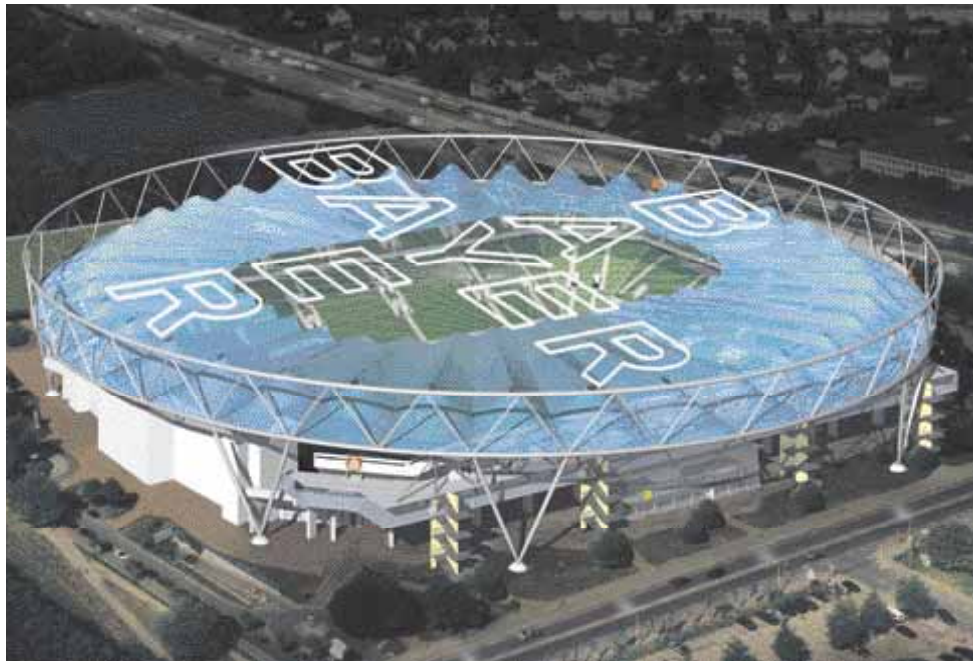
The future BayArena will be covered by a circular, tent-like roof integrating the company's logo. Its 200 meters diameter will make it the world's biggest Bayer Cross.
